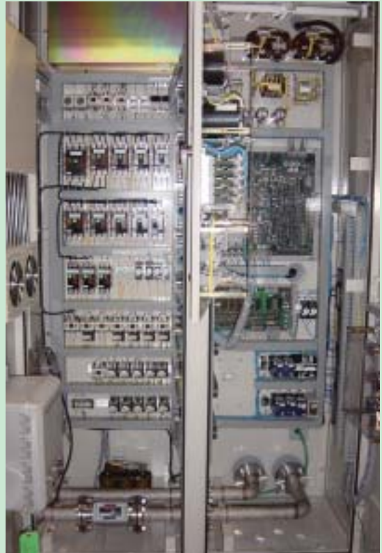
Up-to-date thyristor rectifier control panel
