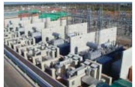
Diode S-Formers for aluminum smelter, 132kV AC/1,330V DC, 85kA each
