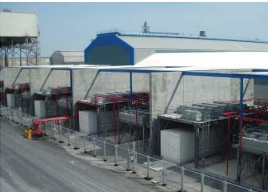
Diode S-Formers for aluminum smelter, 220kV AC/1,580V DC, 72kA each
