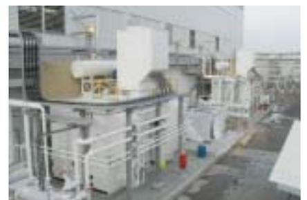
Thyristor S-Formers for chlor-alkali electrolysis, 33kV AC/520V DC, 4 × 30.3kA each
