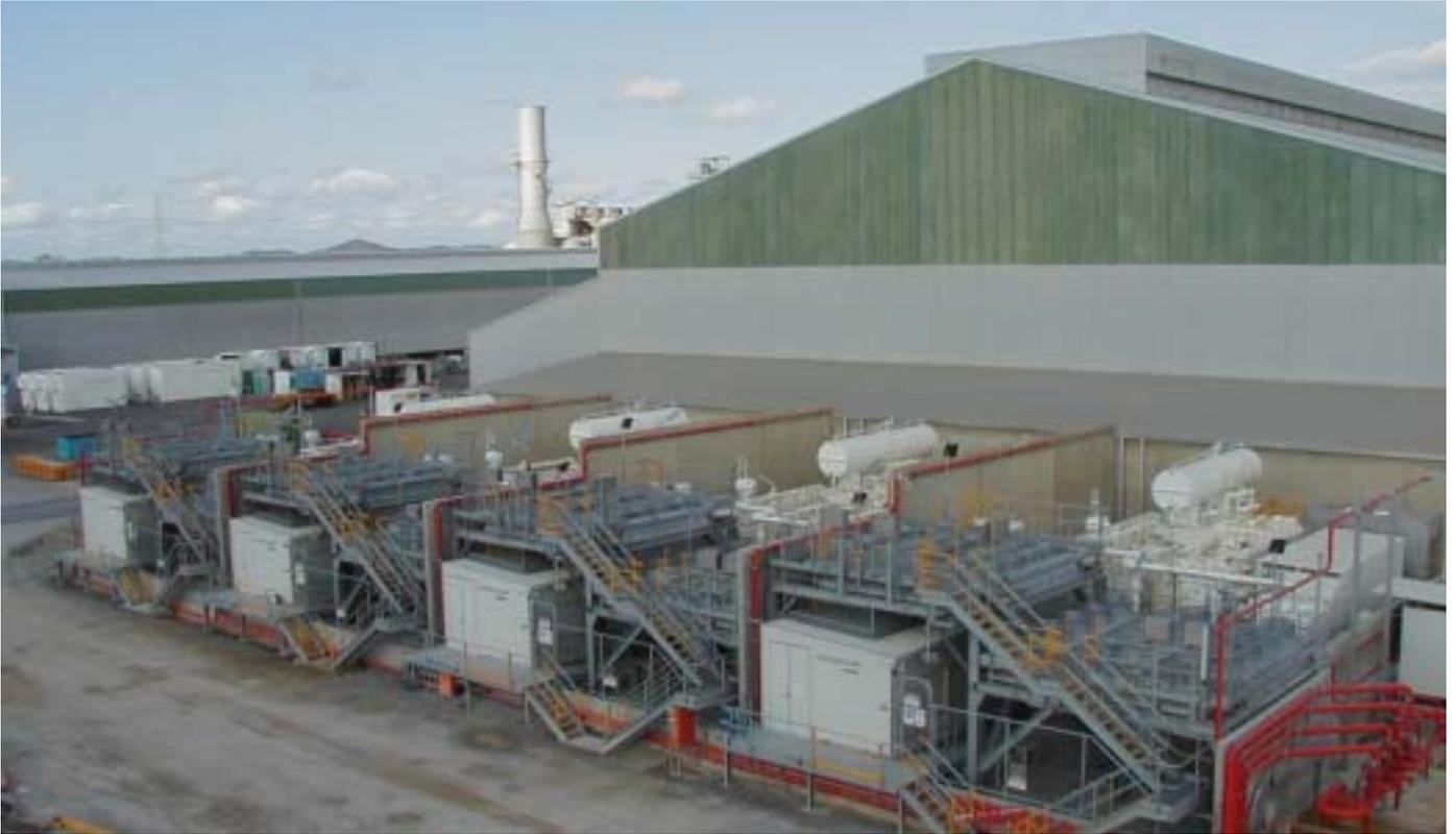
Diode S-Formers for aluminum smelter, 132kV AC/1,450V DC, 82.5kA each
