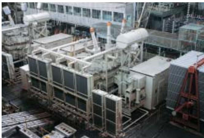
OFAF (forced oil, forced air) cooled transformer and WFAF (forced water, forced air) cooled rectifier
